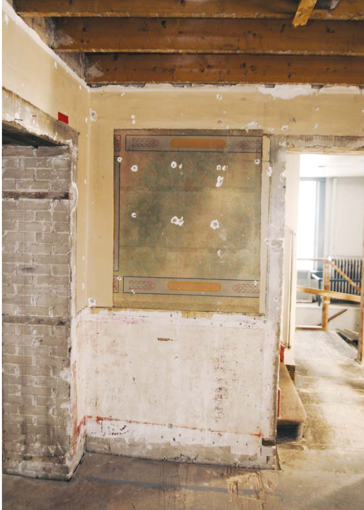
Foyer wall detail.
