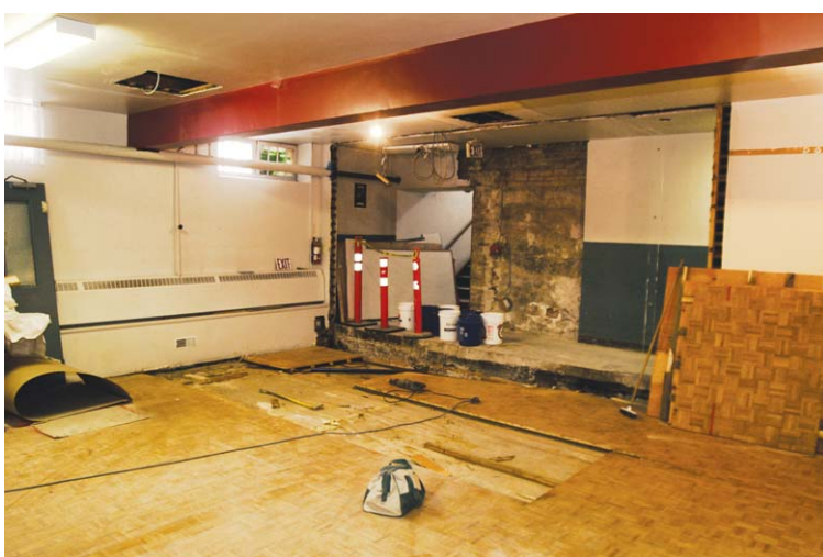
Basement new entrance area.
