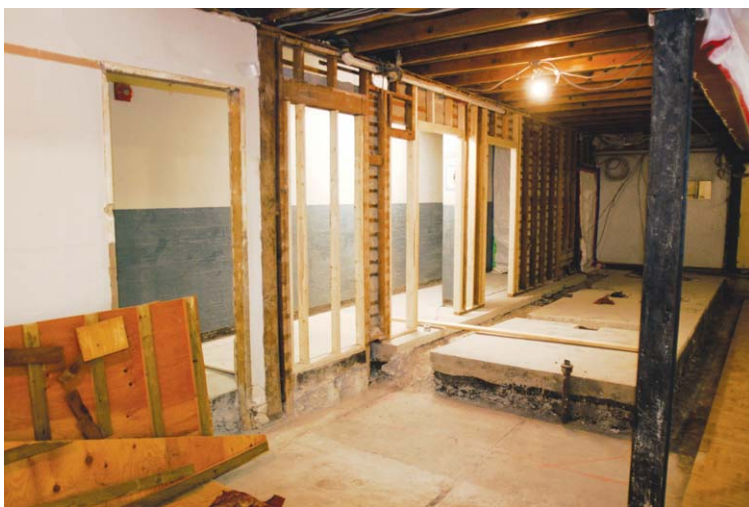
Basement new washroom area.
